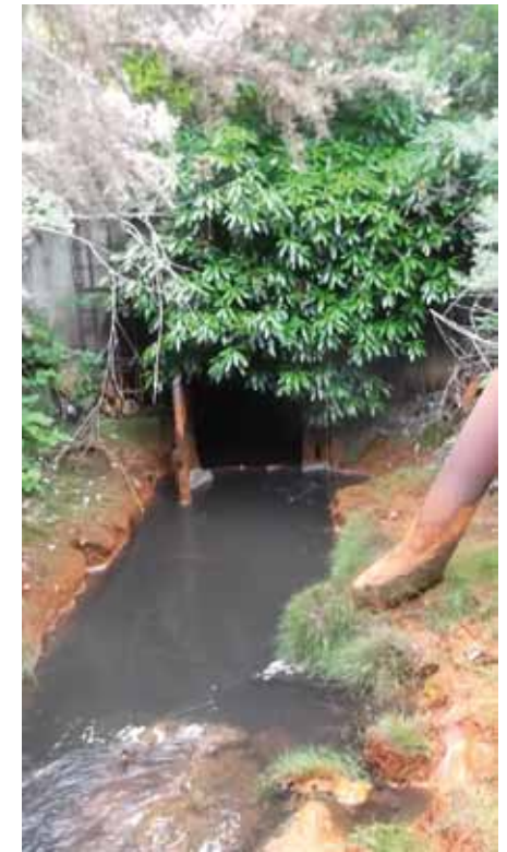
The portal of the Great County Adit today
