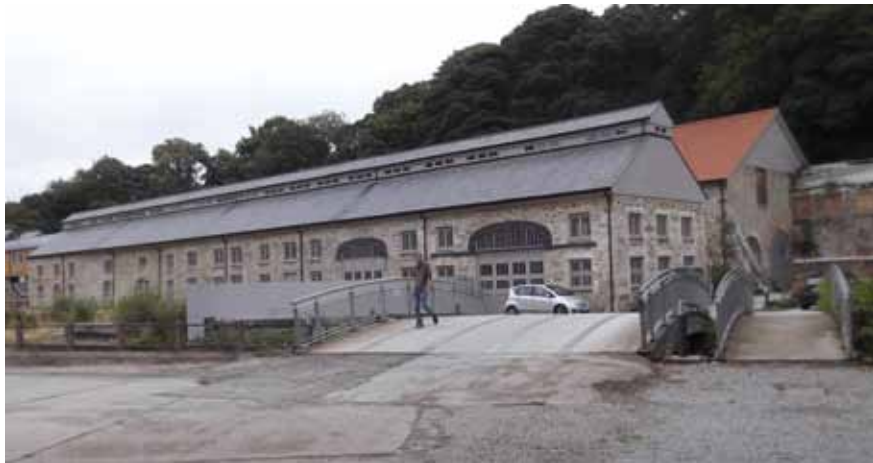
Perran Foundry today
