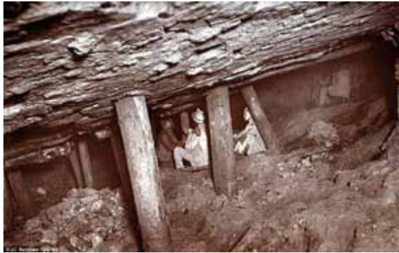
The timbermen cut and installed the props
